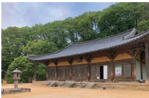
Muryangsujeon Hall of Buseoksa Temple | Yeongju, Gyeongsangbuk-do | 2020 | Korea Heritage Service
